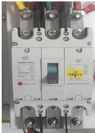
AC inline switch (L1、L2、L3 In-line to AC plastic shell circuit breaker)
